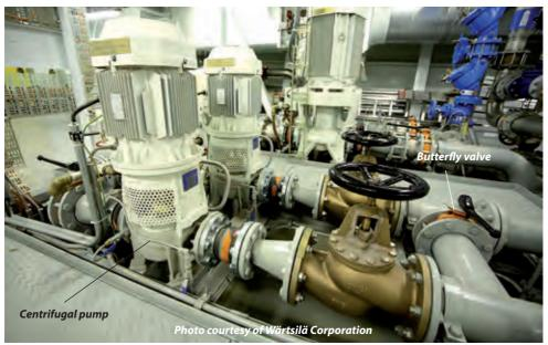
**Centrifugal pump** – It develops its pressure as a result of centrifugal force. Liquid enters the centre of the impeller and flows radially out between vanes. Its velocity being increased by the impeller rotation. It escapes through a discharge pipe at the circumference of the casing.
