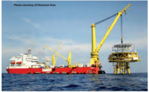
Crane ship SAPURA 3000 placing topside installation
