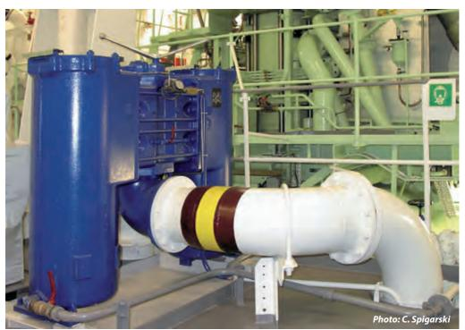
Main Engine fuel oil duplex indicator filter
