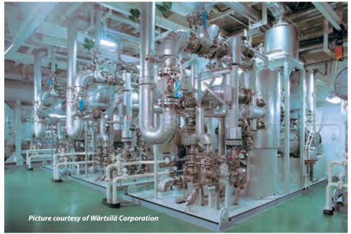
Reliquefaction plant onboard SANHA LPG FPSO
