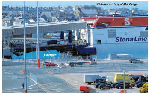
**Double-level linkspan** – If the **ro-ro ferry** has two or more trailer decks, a double level link spans with direct access also to the upper cargo deck saves much time for loading and unloading in port.
